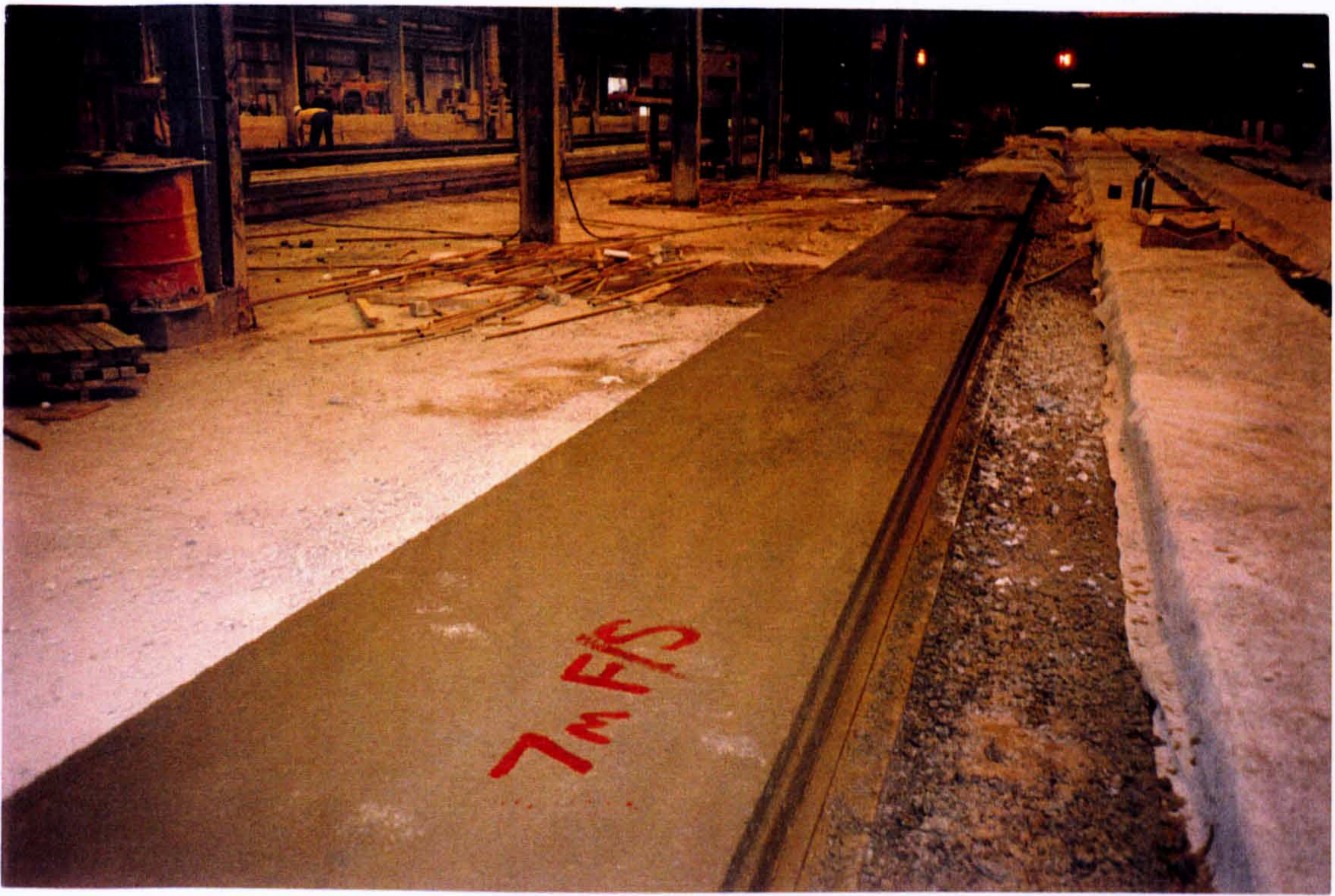
Plate 6-1 Compaction of the three batches at the preliminary trial
