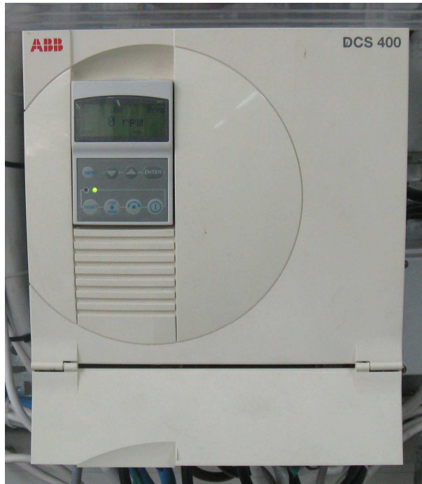
Figure 4.40: DC drive converter
