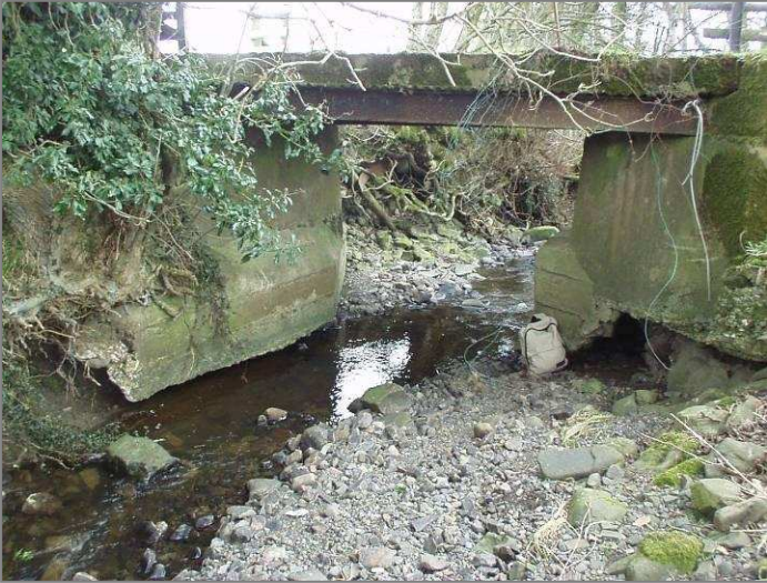
Figure 2.10 (a) Exposed bridge buttresses and (b and c) steep banks due to channel incision in the Upper Pontbren subcatchment.
