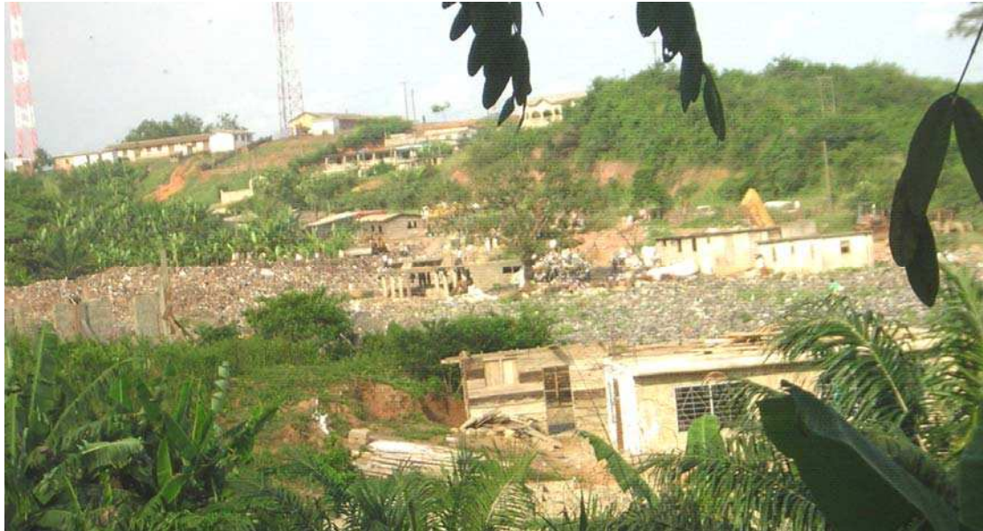
Figure 5.18: The final disposal ground near Mpinstim is a poorly managed facility
