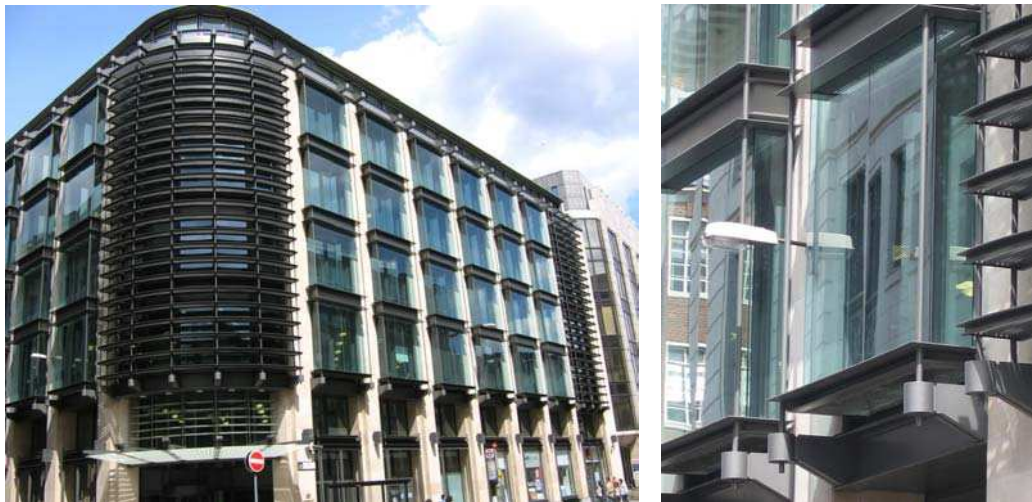
Figure 2.28 Facade view of the main entrance on Cannon Street and close view of a Shaft Box Double Skin Facade module. Photos: M. Hernandez T (2006).
