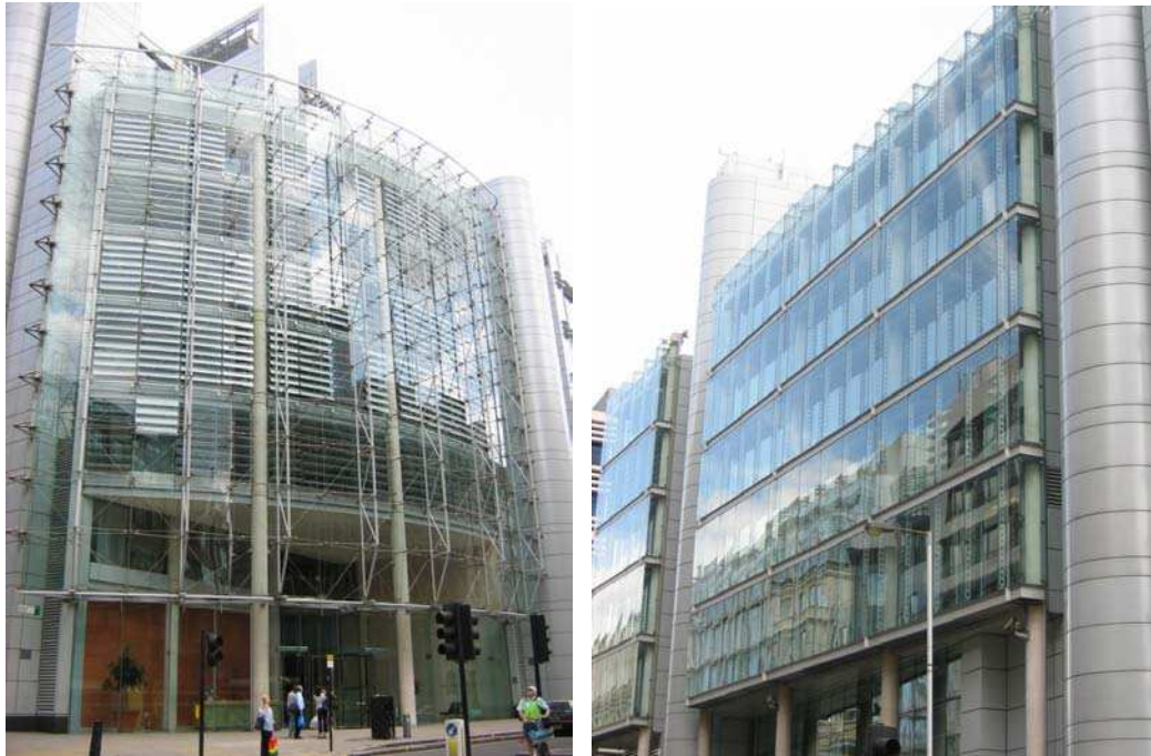
Figure 2.31 View of the DSF over the main entrance at Finsbury Pavement and view of the Corridor DSF facing Finsbury Pavement. Photos: M. Hernandez T (2006).
