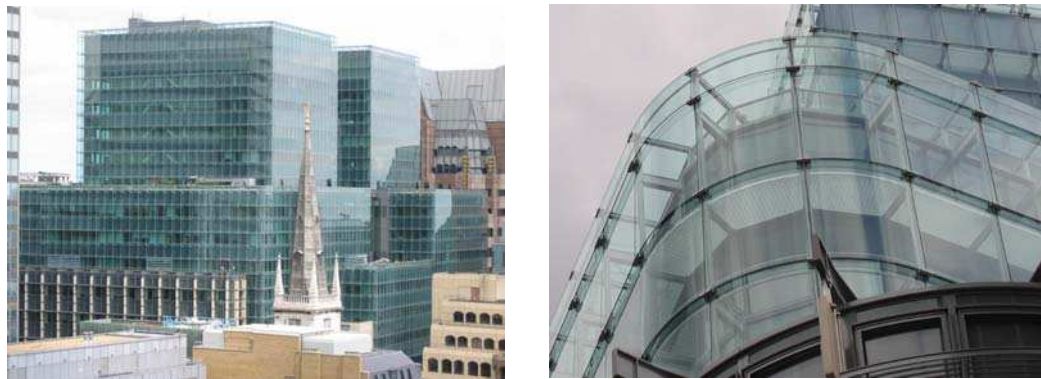
Fig. 2.25 General view of the building from the south west and close view of the North-east facing corner Double Skin Facade. Photos: M. Hernandez T (2006).
