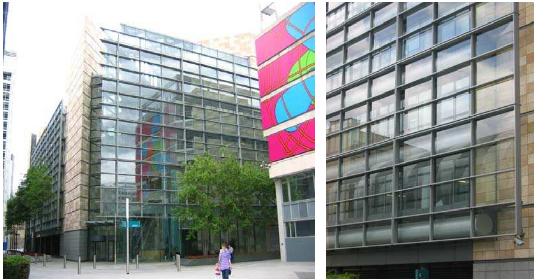
Figure 2.26 View of the south-east main entrance from Triton Square and close view of the north facing Double Skin Facade. Photos: M. Hernandez T (2006)
