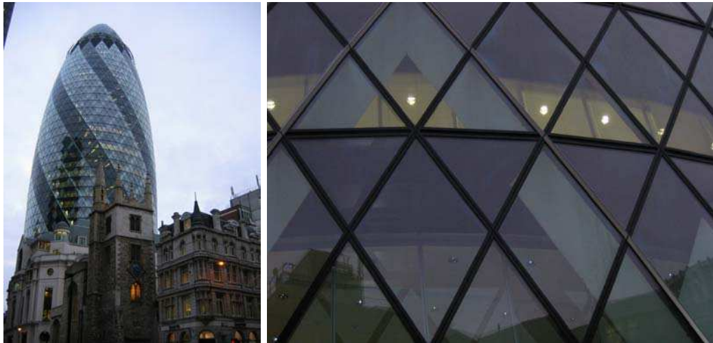
Figure 2.37 General view of the building from St Mary Axe and close view of the Double Skin Facade. Photos: M. Hernandez T (2006).
