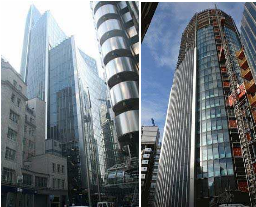
Figure 2.40 General views of the building from North-west and South-east corners. Source: MERO-SCHMIDLIN (UK) PLC. http://www.merouk.co.uk/curtainwalling/50001limest_construction.htm
