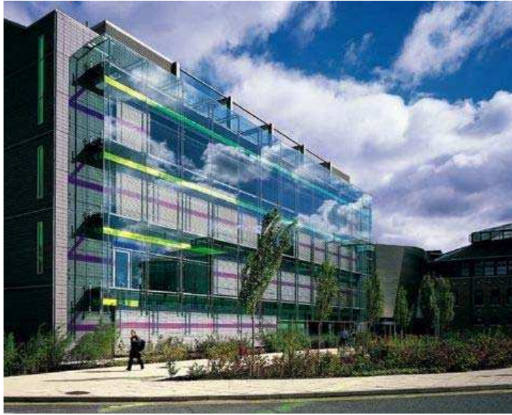
Figure 2.34 General view of the building Source: www.wilkinsonseyre.com Photo: Nick Wood.
