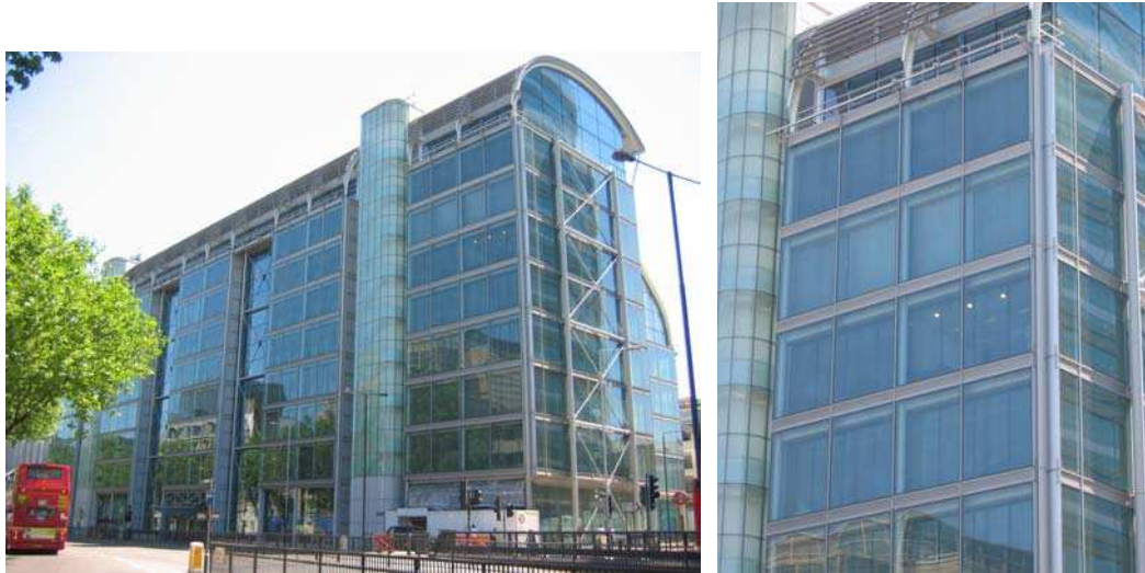
Figure 2.33 General view of the building's north facade from Houston Road and close view of the Corridor type Double Skin Facade. Photos: M. Hernandez T (2006).
