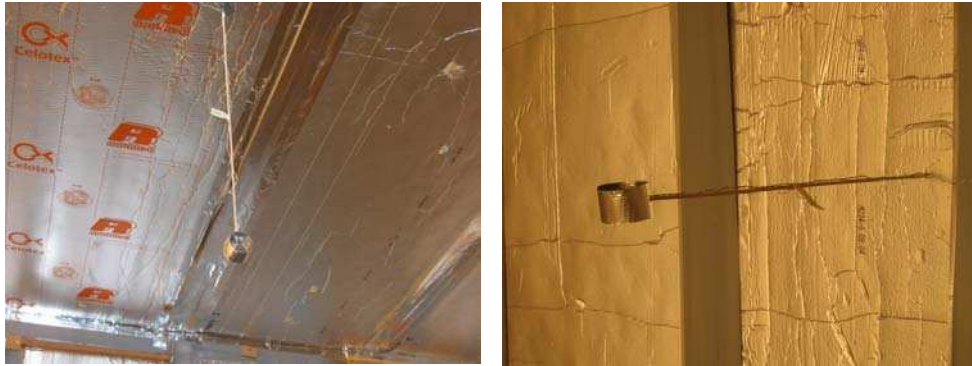
Figure 4.16 Shielded K-type thermo-couples placed inside the chamber room.
