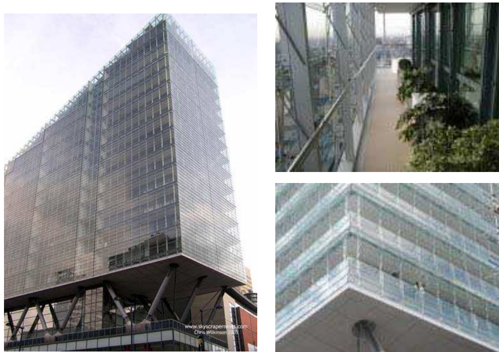
Figure 2.39 General view of the building and close views of the DSF. Sources: http://www.skyscrapernews.com , Photo: Chris Wilkinson, 2005. http://www.merouk.co.uk/structures/2002deansgate.htm
