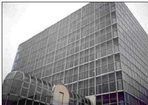
Figure 2.14 The Hooker Building southeast Double Skin Facade, 1980. (Harrison, 2003) http://www.architecture.uwaterloo.ca/faculty_projects/terri/ds/hooker.pdf
