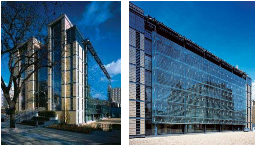
Figure 2.32 General view of the building from the South-east and general view of the south facing Multi-story Double Skin Facade.
