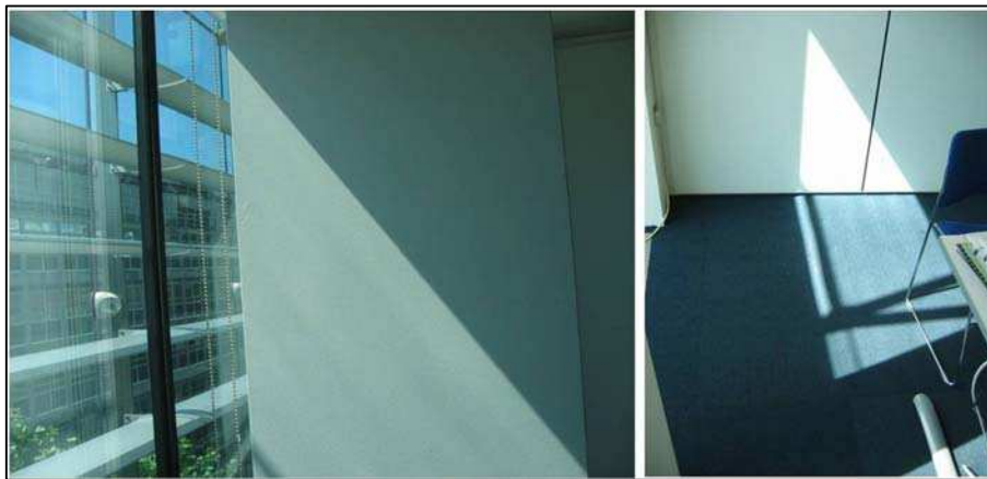
Figure 7.23 Direct radiation hitting inside the room on walls and floor as the shading devices were not totally able to shield efficiently part of the inner facade.
