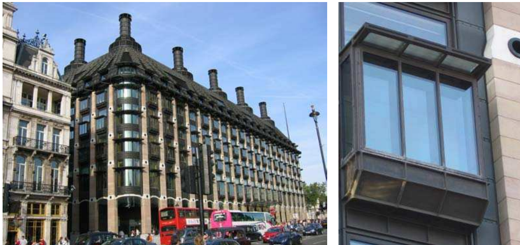
Figure 2.36 General view of the building on Bridge Street and close view of the Shaft-Box Double Skin Facade module. Photos: M. Hernandez T (2006)
