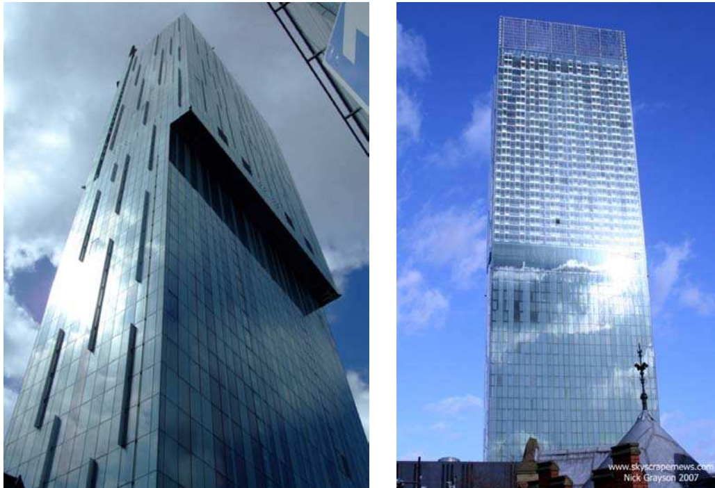
Figure 2.41 General views of the building. Sources: http://en.wikipedia.org/wiki/Image:Beetham_tower.jpg http://www.skyscrapernews.com/buildings.php?id=132 Photos: Iain Dickinson (2006), Nick Graysen (2007).
