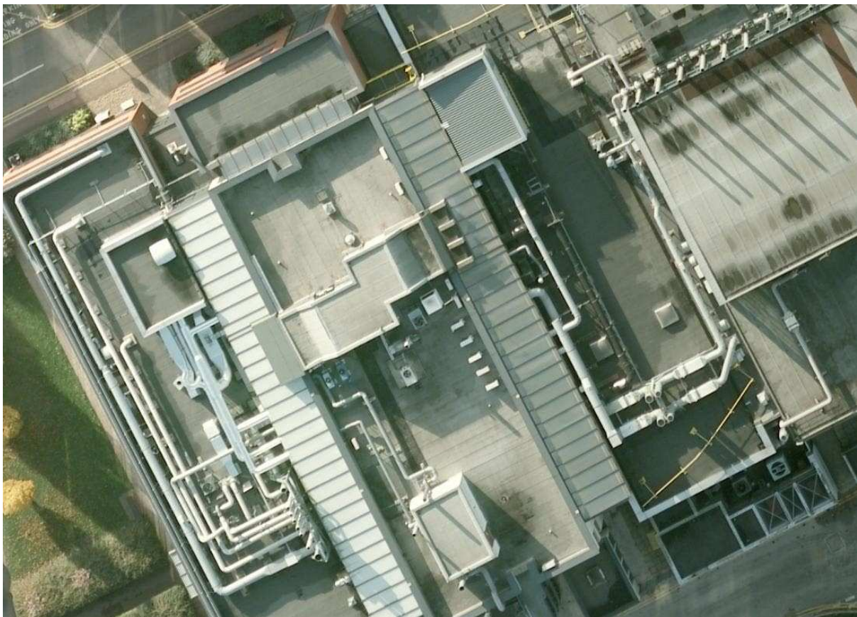
Figure 74. Subset of an UltraCam D image over Nottingham test site representing one of the chemical engineering buildings of increased roof complexity
