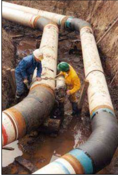
Figure 1.2: Construction on pipeline (adopted from www.ncl.ac.uk )
