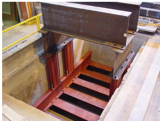
Figure 4.2. Testing frame in the pit
