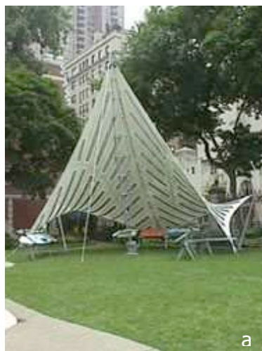
Fig. 2-35a Membrane structure with PVs for the "Under the Sun" Exhibition, FTL Happold Fig. 2-35b Scale model of the project
