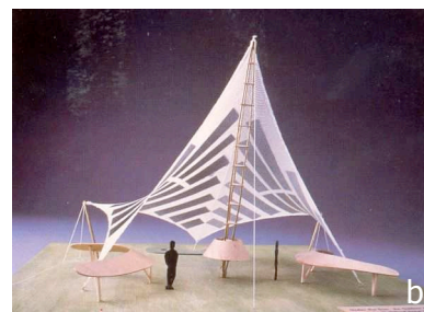
Fig. 2-35a Membrane structure with PVs for the "Under the Sun" Exhibition, FTL Happold Fig. 2-35b Scale model of the project
