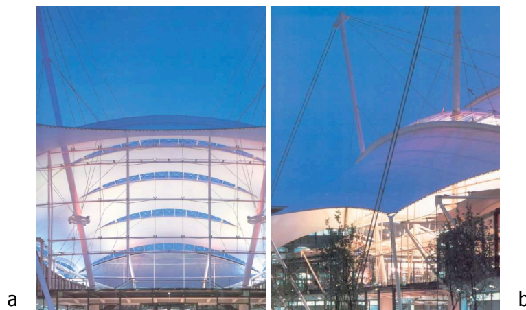
Fig. 2-32a & b Amenity Building of the Inland Revenue Centre, Nottingham.
