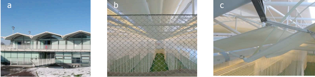
Fig. 3-10a Main façade National Cricket Academy. Fig. 3-10b Interior view of playing area. Fig. 3-10c Fabric louvres.
