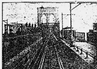
ENTRANCE TO COVERED WAY ON NEW YORK SIDE.
