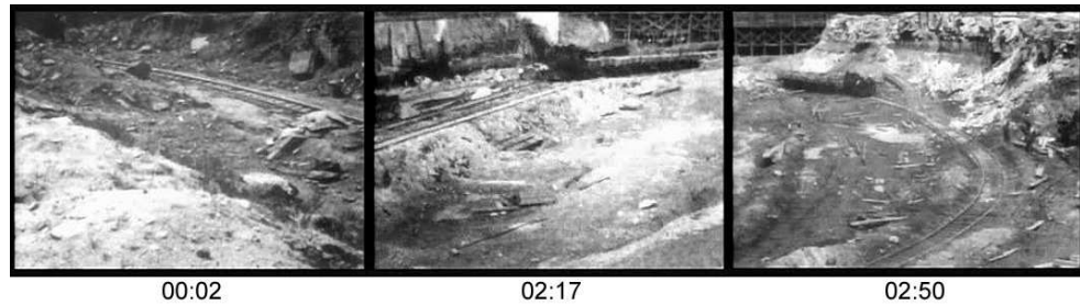
Fig. 5.6 Frames from Pennsylvania Tunnel Excavation (AM&B, 1905).
