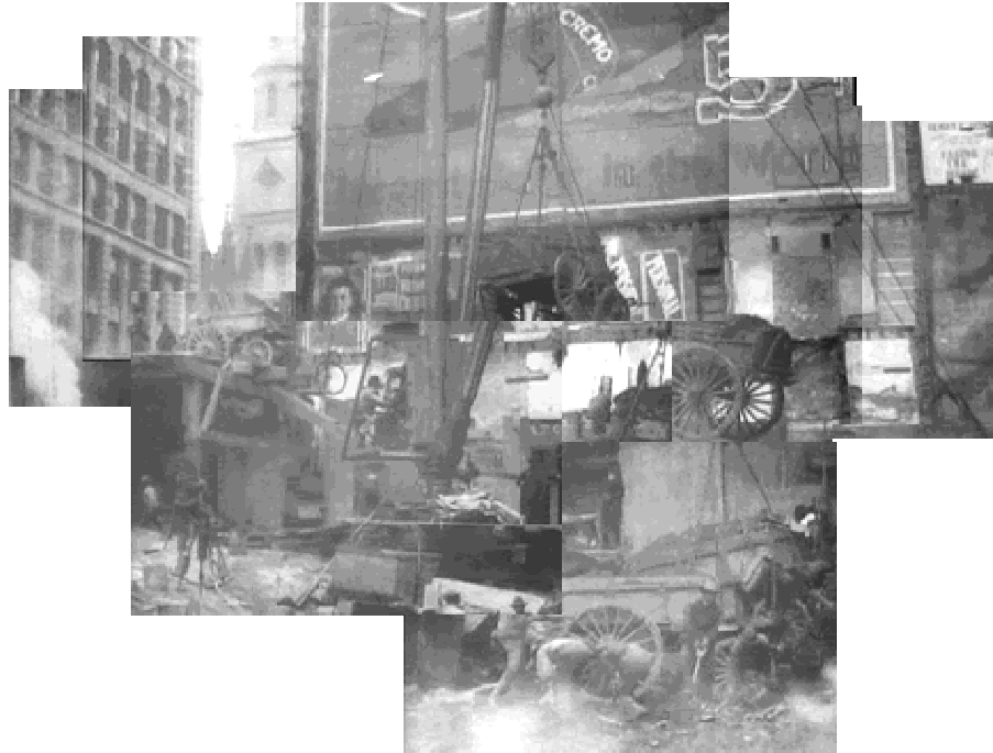
Fig. 4.5 Composite of frames from Excavating for a New York Foundation (AM&B, 1903)
