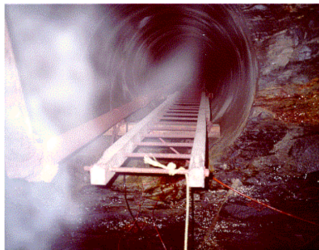
Figure 5-6: Diesel fumes upcasting a ventilation shaft
