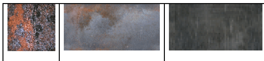
Figure 5.12: Watertube boiler texture images
