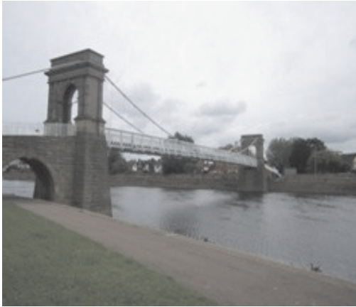
Fig. 8. Wilford bridge over the River Trent in Nottingham, UK.
