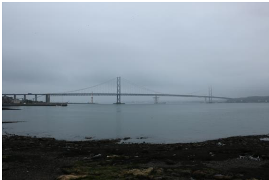
Fig.1 The Forth Road Bridge in Scotland is over 50 years old and has a main span of 1006 metres long. This bridge is used as a test-bed for GeoSHM project
