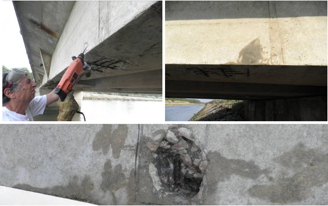
Figure 11. Window to inspection the condition of reinforcement bars.
