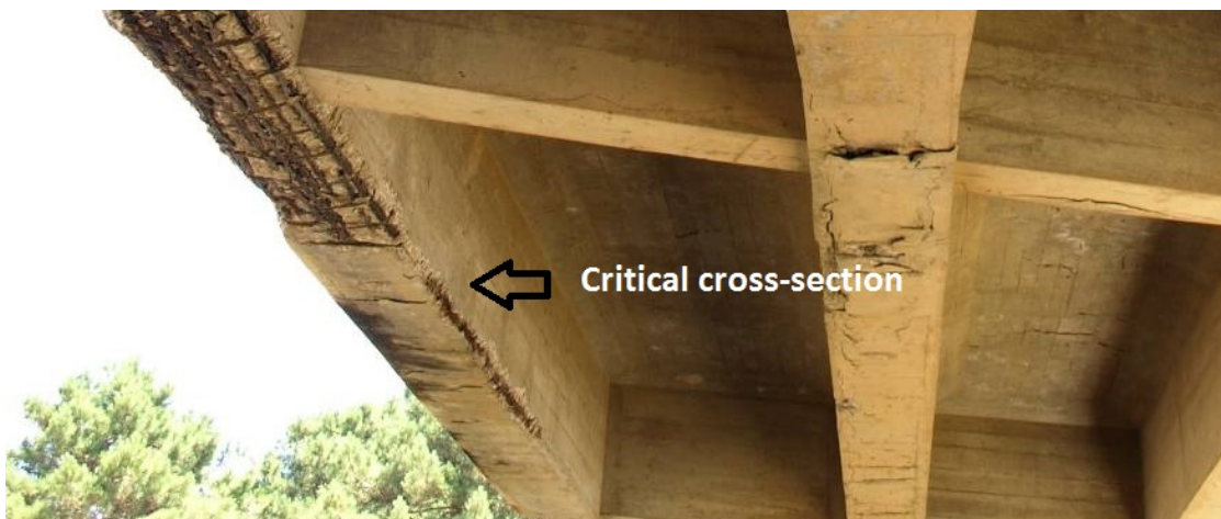
Figure 10. Condition state of the critical cross-section.
