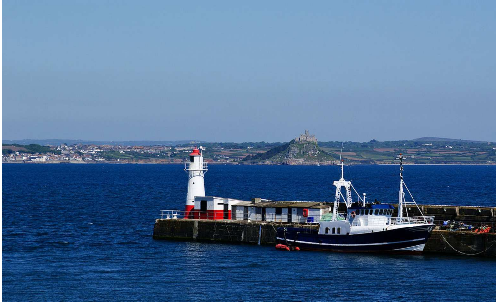
Figure 2. A view to the north-east, from Newlyn Harbour to St. Michael's Mount, showing the lighthouse and Tidal Observatory to its right, both painted red and white. The white GPS antenna on top of the lighthouse platform can be clearly seen. Photograph taken in 2010. A Wikimedia Commons image. 451x272mm (72 x 72 DPI)
