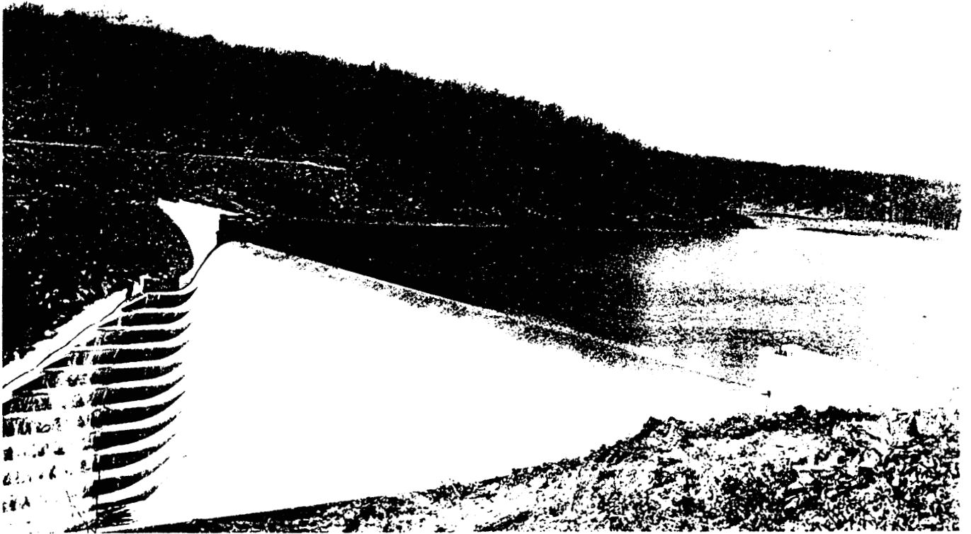
Liberty Dam, located on the North Branch of the Patapsco River, sends raw water by gravity to the Ashburton Filtration Plant.
