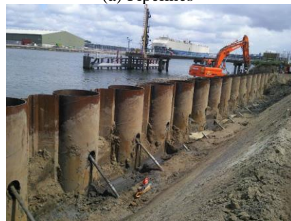
(b) Sheet Piles 7
