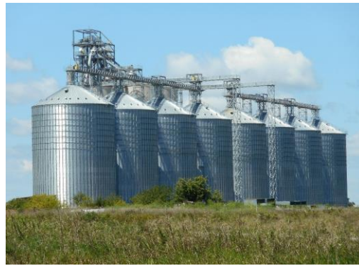
(a) Steel silos 3
