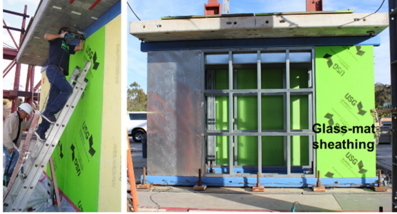
(a) Glass-mat sheathing installation
