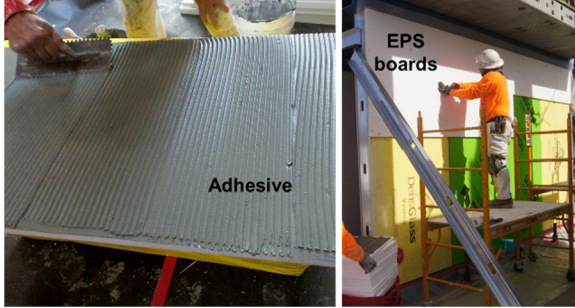
(b) 1" thick Expanded Polystyrene (EPS) foam boards attached using cement adhesive
