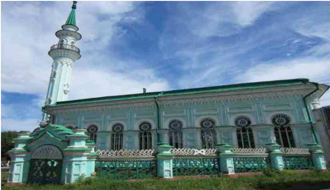
Figure 5: The Acem Mosque exterior.
