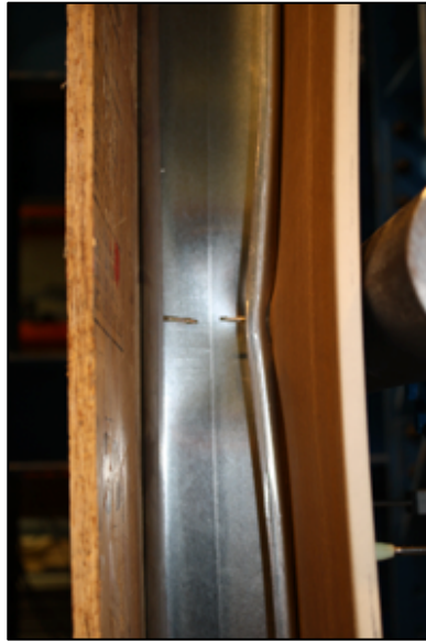
(b) detail of (a) at point of lateral load application, connection damage limited
