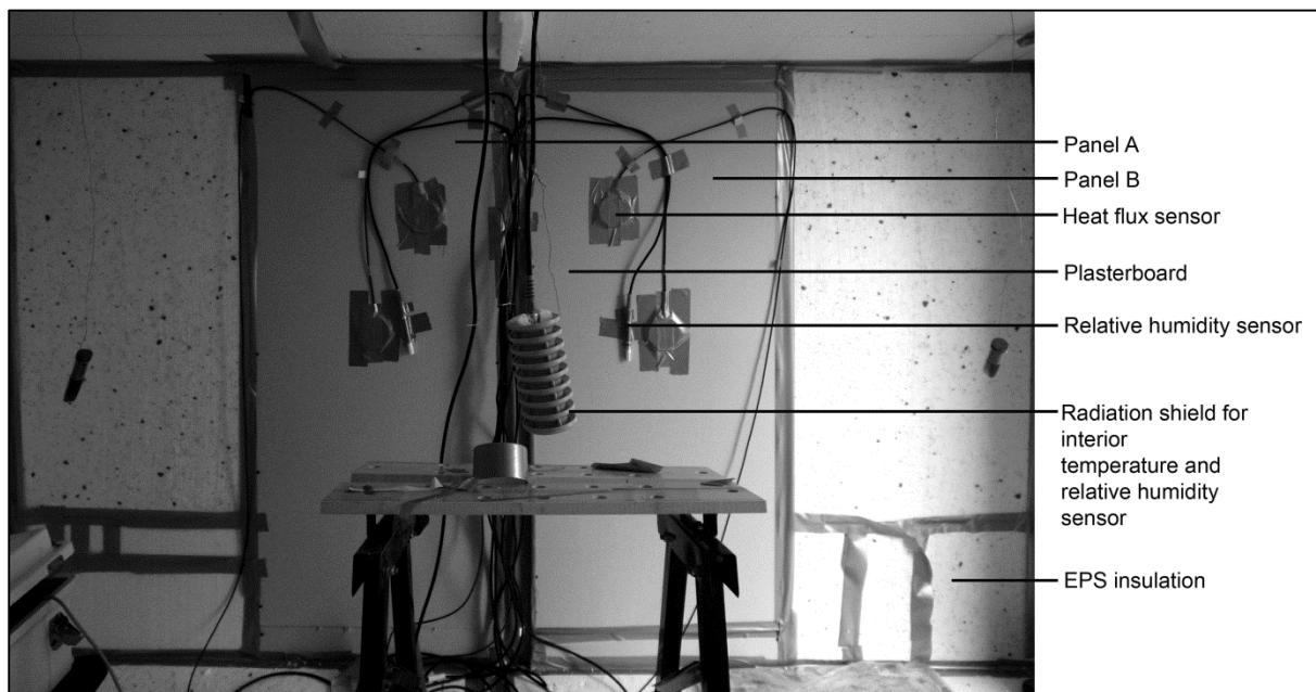
Fig. 7. The installation of the surface lining and the sensors.
