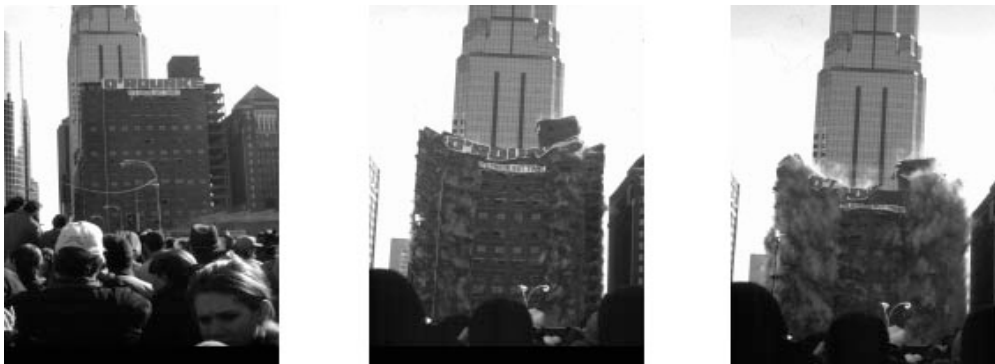
10; Kansas City demolition of a skyscraper
