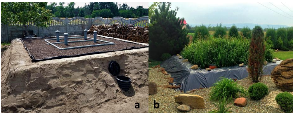
Figure 4 LECA-based Vertical Flow Constructed Wetland before (a) and after (b) commissioning. LECA has become one of the most commonly applied substrates for small scale, domestic CWs systems, which account for roughly 3000 units in Poland alone ( personal communication ). (Photo. F. Bydalek/ Ecoverde Engineering Office, Poland).
