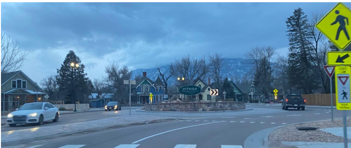
Figure II-C: 5-Way Intersection Roundabout in Colorado Springs, View from S. Tejon St.
