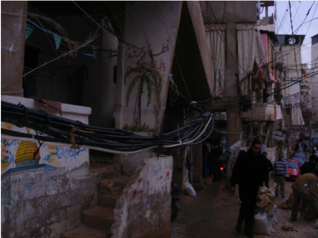
Figure 4.27: Bourj Al Barajneh Refugee Camp Courtesy of Tom Charles, Contributor at Jadaliyya.com 326
