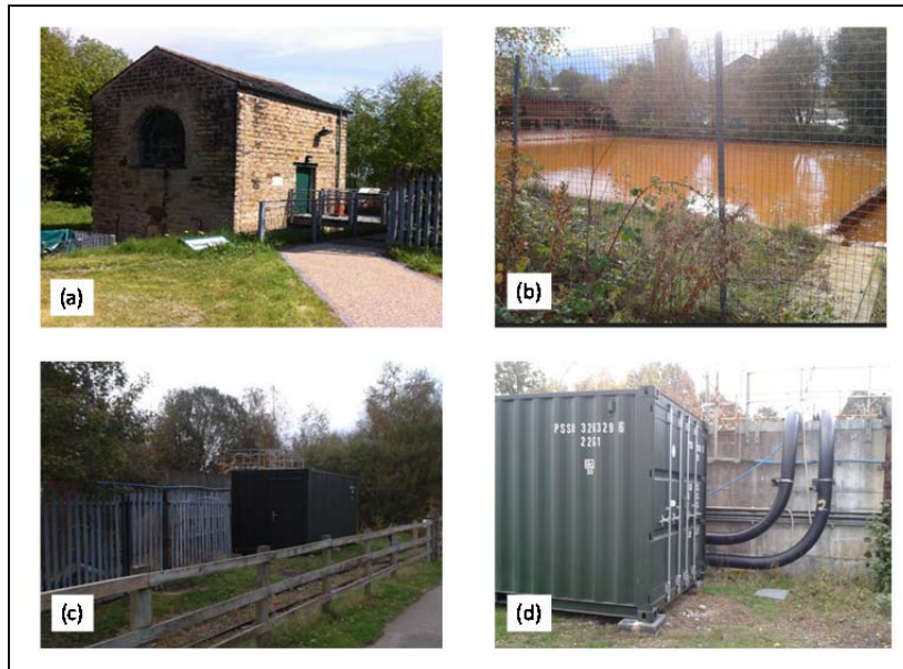
Figure 3: Main components of the system, Inman shaft building heated by the heat pump (a), the lagoon (b), plant housing container (c) and the container with the main two pipes that pump the water from the coal mine (d).
