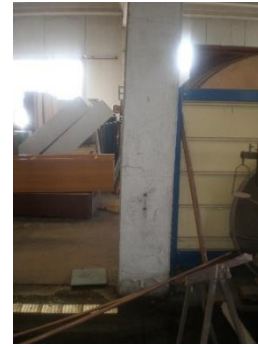
Figure 4. Rotation of the columns along the X direction after the event on May 29 th
