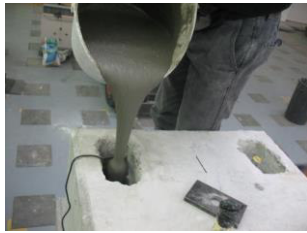
Figure 3. Cast of grout in the beam holes
