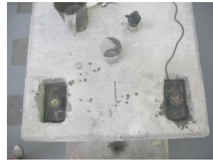
Figure 4. Dowels restrained at the top of the beam by means of steel plate, nut and washer
