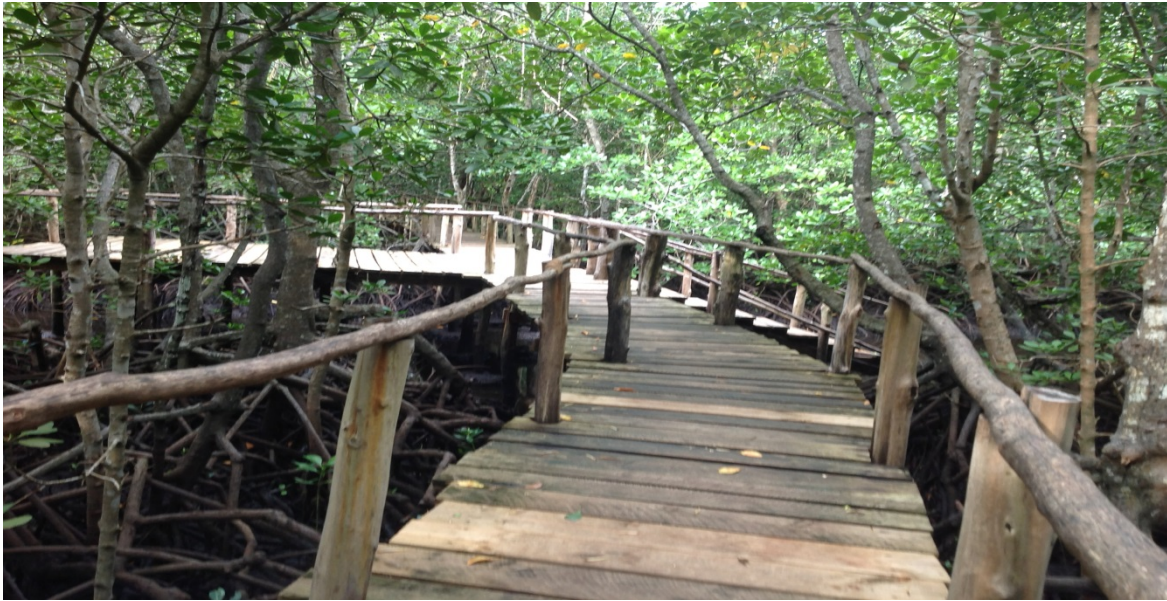
Plate 2 Pete-Jozani mangrove boardwalk. Source: field survey, 2013
