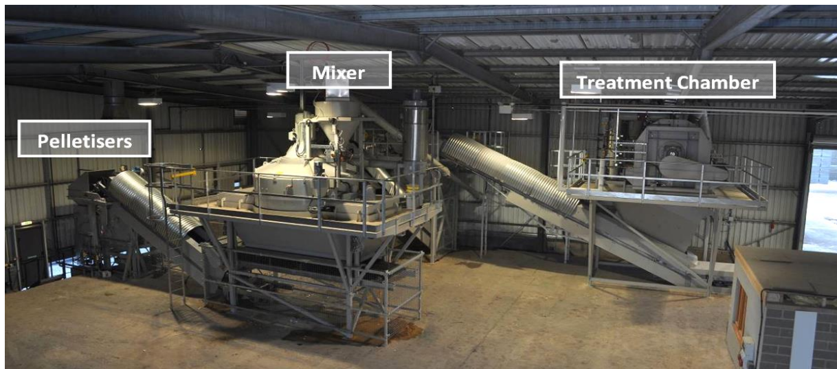
Figure 5. The newly commissioned plant
