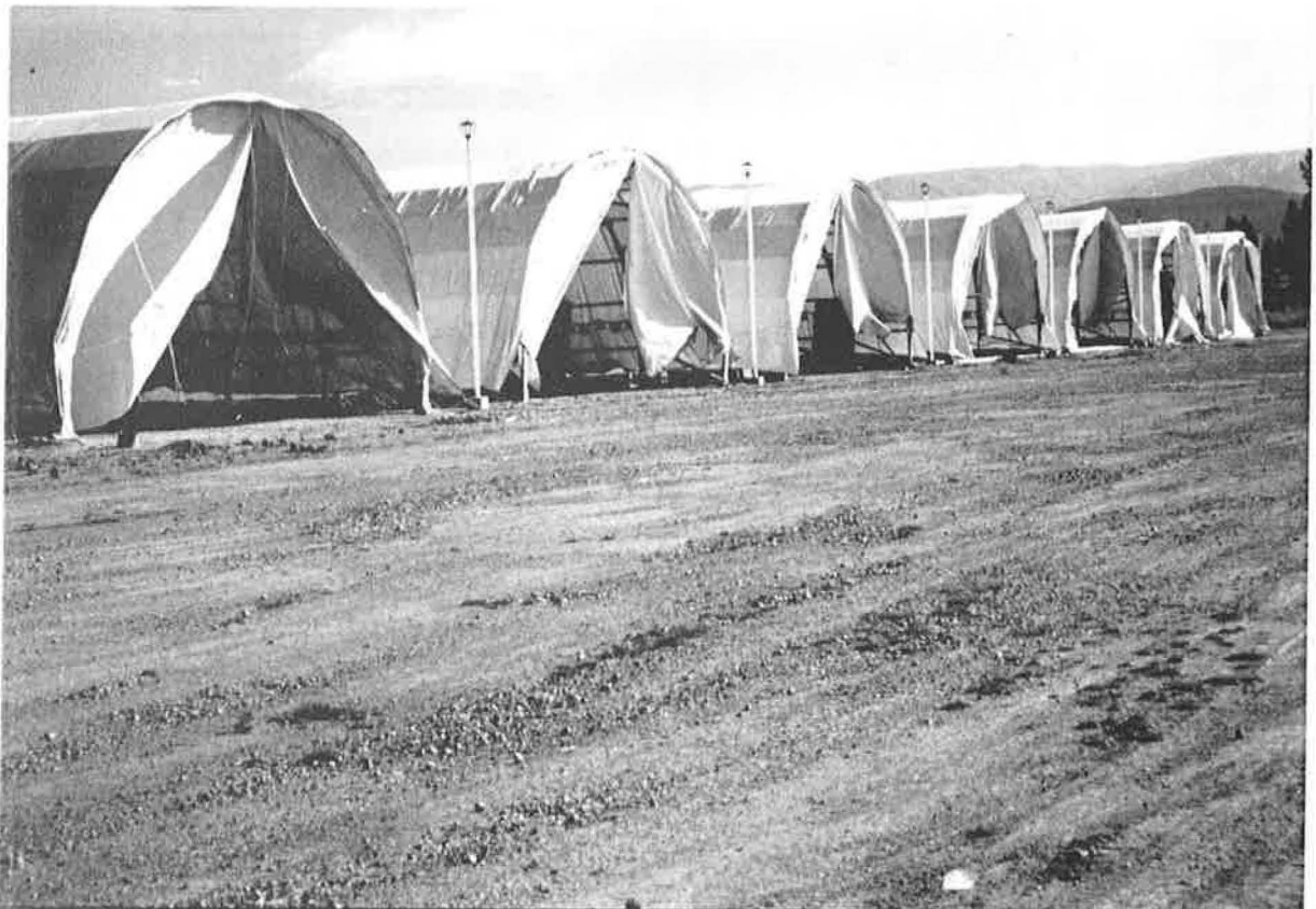
Completed stores with cladding, Ecuador
