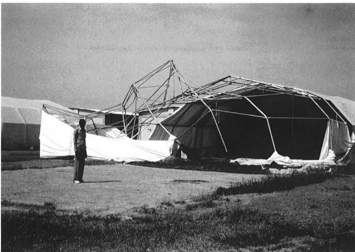
Failure of plastic-clad building caused by wind forces. Mali
