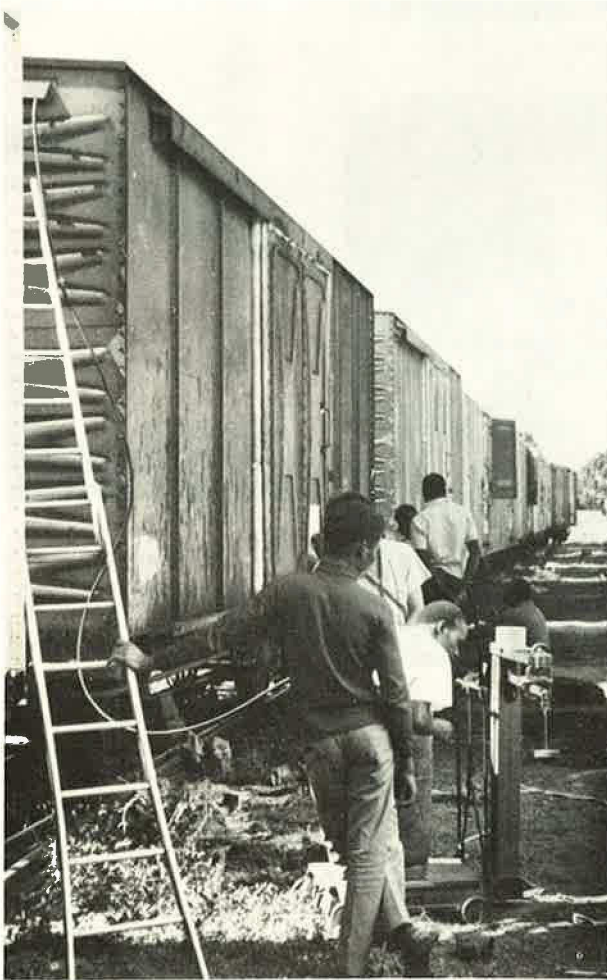
Fig. 4. The introduction of methyl bromide through tubing which has been temporarily placed through the ventilators at the end of the truck. Note also the gas cylinder upon weighing scales.
