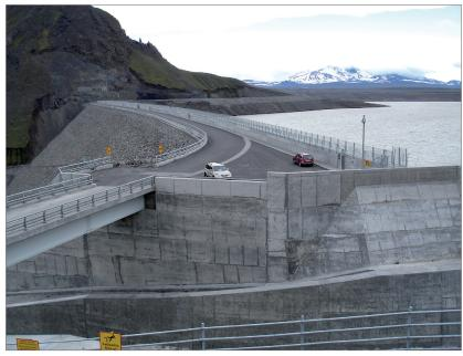
Figure 48: Blackwater dam, Scotland, built 1905-08, 27m high, 914m long, 20 MWh/a. Main dam (of 2) of Blackwater Hydroelectric Project, powering British Aluminium smelter (now Rio Tinto Alcan).
