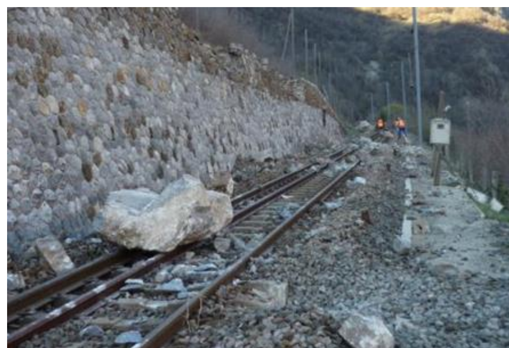
Fig. 2 Falling Rocks blocked the railway in Bourg St Maurice France, May 2015.
