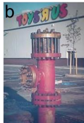
Figure 3 – (a) Geothermal drilling in Newcastle upon Tyne in 2011 (b) Geothermal wellhead at the Southampton scheme. This photo was taken during maintenance work; usually the wellhead is encased in insulation and is even less conspicuous.
