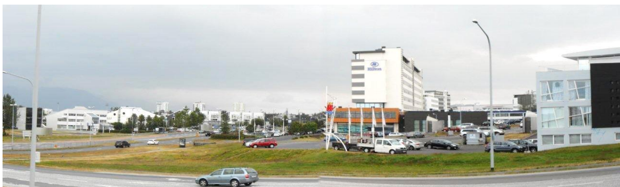
Figure 25 – Geothermal wellfield in Reykjavik. The wells are in inconspicuous cabins about the size of bus shelters
