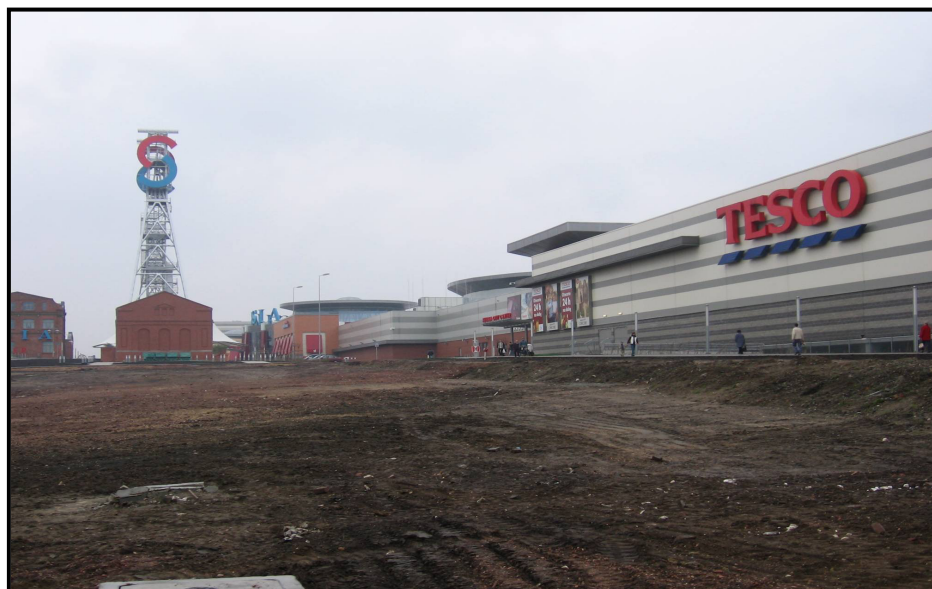
Figure 2. Redevelopment of the Kleofas mine site, Katowice, Poland (photo by © David Banks).
