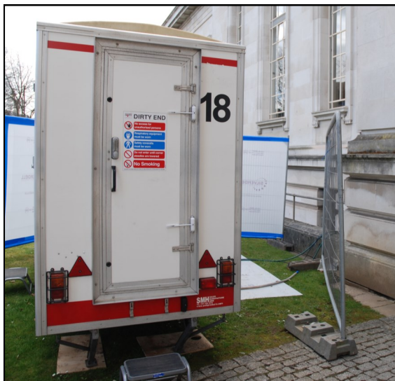
Fig. 10. Typical trailer-style decontamination unit used by asbestos contractors. This may be placed inside a storage area if space allows, although here it is show placed external to the building. National Museum of Wales decontamination work 2013.
