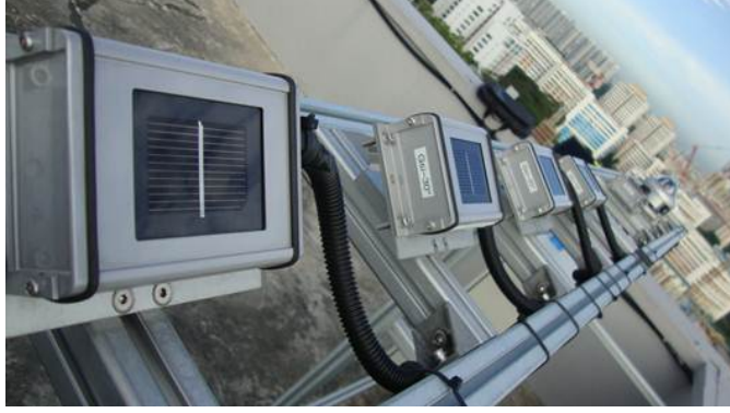
Figure 1: Photograph of the irradiance measurement station located on the rooftop of the Solar Energy Research Institute of Singapore (SERIS).
