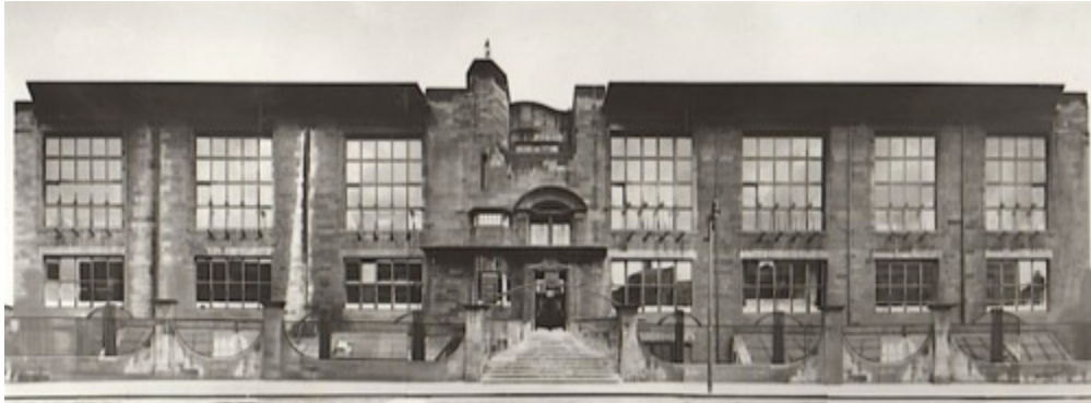
Fig. 1, North façade of Charles Rennie Mackintosh's The Glasgow School of Art, ca. 1910. Photograph. The Glasgow School of Art. [return to text]
