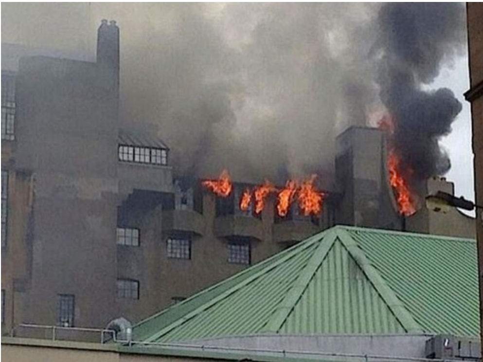
Fig. 9, Flames coming out of the Hen Run on the south façade. Public Domain. [return to text]
