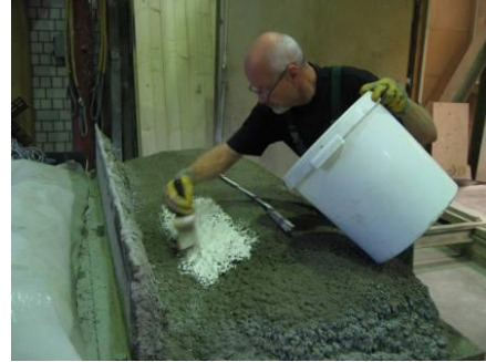
Figure 6: Applying the sprayable waterproofing membrane by brush as confirmed by manufacturer
