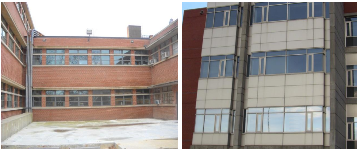
Figure 3: Two building façades for multi-step stereo camera calibration experiments
