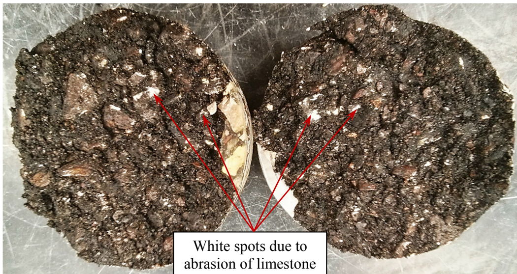
Fig.10 White spots due to abrasion of limestone aggregates on shear failure surfaces of asphalt concrete
