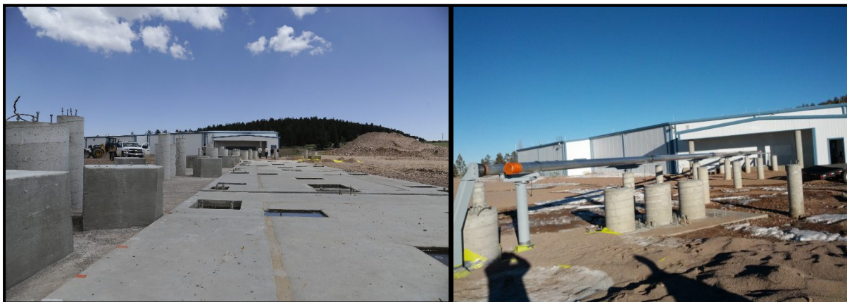
Figure 6: A view along the west array arm of the interferometer looking toward the beam combining facilities. At left are four of the telescope and enclosure foundations are shown together with the beam relay and vacuum can piers running along the left-hand side of the photo. At right, the foundations have been covered to protect them from heavy equipment, and installation of vacuum pipes has begun.
