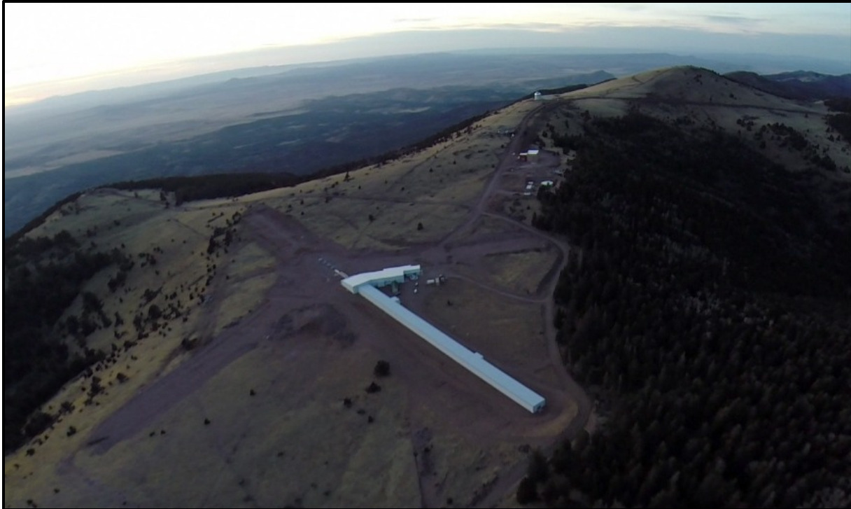
Figure 1: Overview of the Magdalena Ridge at 10,500 feet looking northwest. In the foreground is the beam combining facility and the completed array arms for the MRO interferometer. Far in the background is the 2.4m fast-tracking telescope. The location of the NRAO EVLA is on the plains below in the upper left of this image. (Picture courtesy of Bob Martin, Albuquerque, NM).
