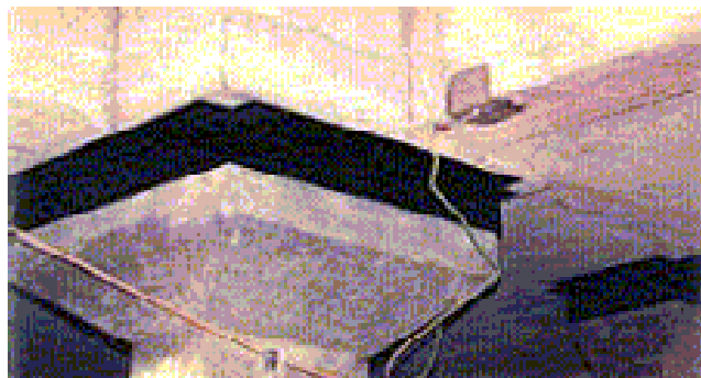
Figure 2.5: One of the natural rubber bearings isolating Glasgow Concert Hall (courtesy of Silvertown UK Ltd, Burton-upon-Trent, UK). The bearings are located in the basement on top of concrete columns that support the building.
