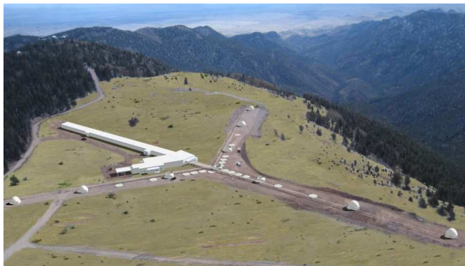
Fig 1: An artist’s impression of the Magdalena Ridge Observatory Interferometer when fully deployed. In this figure the 10 telescopes are in their highest resolution configuration which gives a maximum baseline of ~340m. The long delay-line building to the left points roughly east.
