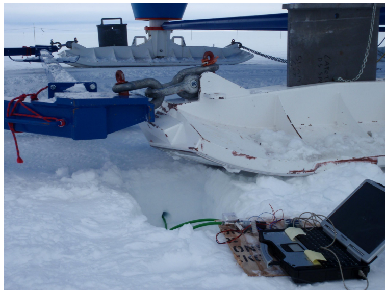
Figure 3.15: Opportunistic pressure bulb testing was conducted during module moves.
