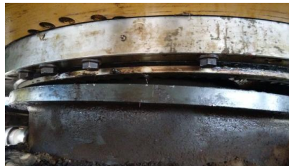
Gambar 7. Proses Disassembly 2 Pelepasan Bolt Upper Structure
