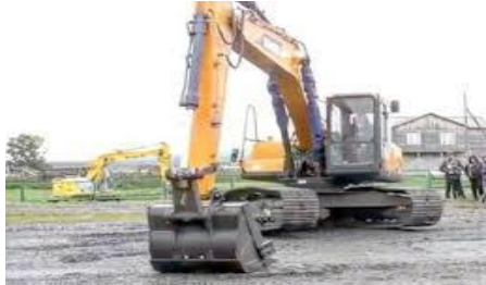
Gambar 11. Gerakan Jack Swing Excavator
