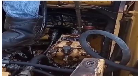
Gambar 6. Disassembly 1 Hose Swing Motor
