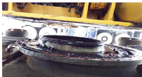
Gambar 8. Proses Disassembly 3 Upper Structure
