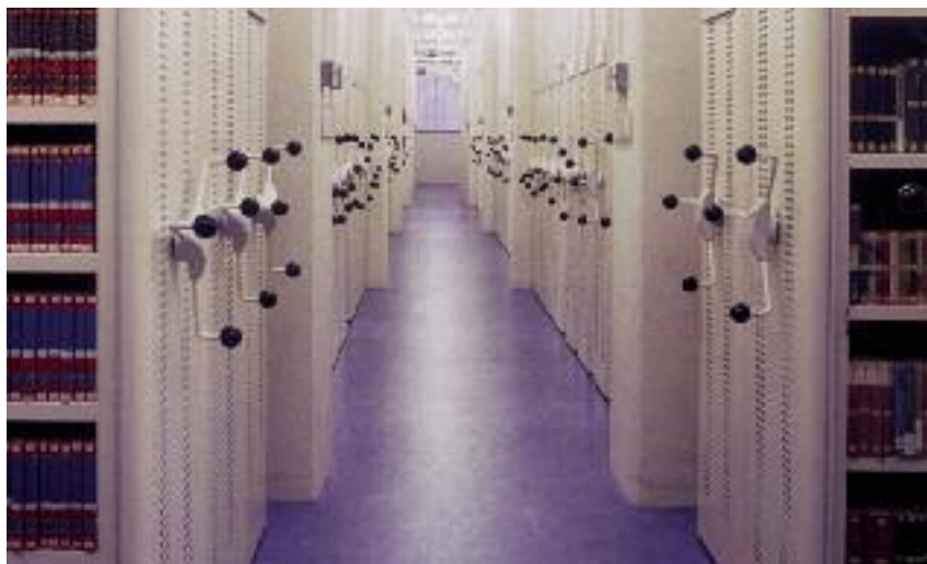
The Library makes extensive use of mobile stacks to maximise its storage capacity; each of these stacks contains several tons of books but can be moved easily thanks to sophisticated gearing.
