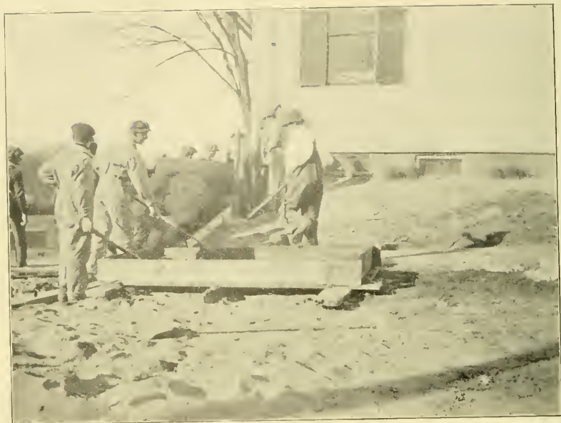
CONCRETE WALL. Made by Pupils in Walpole High School.
